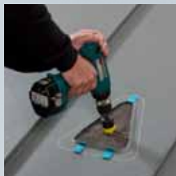
Loch \varnothing 35mm mittig bohren
